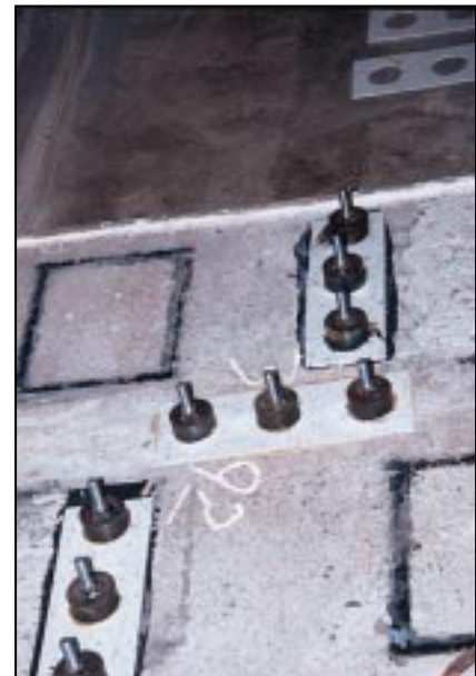
Figure 1. Steel discs glued to 2-inch-diameter plugs of vinyl composition tile were later pulled off to measure the strength of adhesives bonding the tile to concretes with varying water-vapor emission rates.
